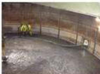
Photo of cleaning sludge From tank bottom
