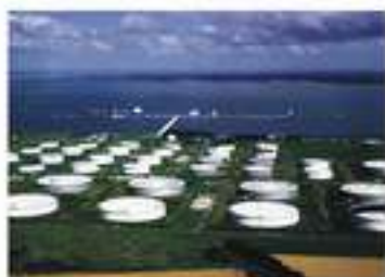
Photo of oil tanks
